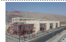
Iraq: substation facilities
